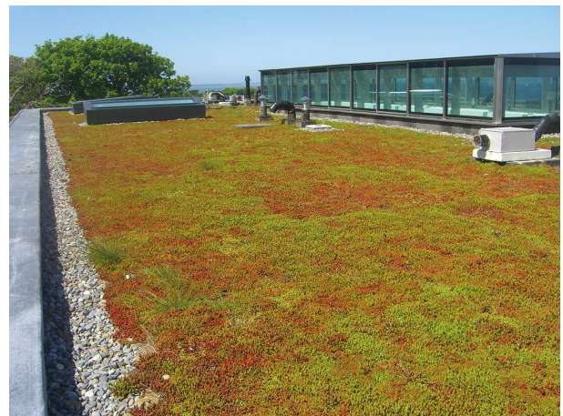
Figure 6; Extensive green roof
