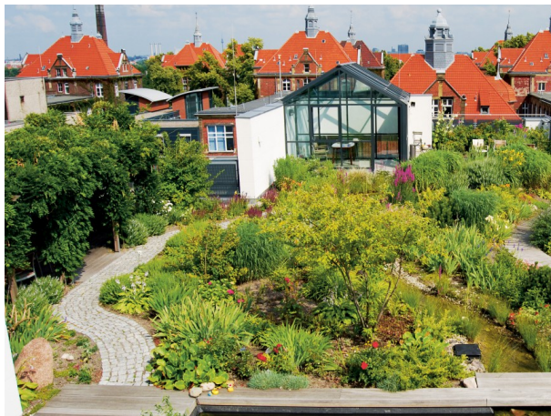
Figure 7; Intensive green roof
